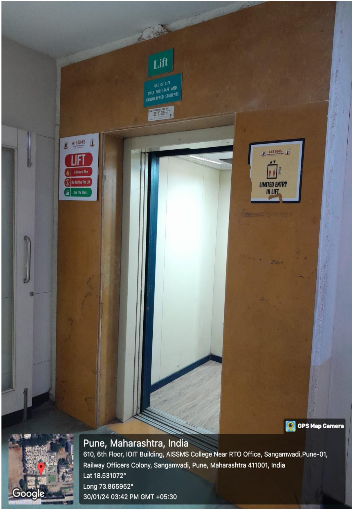
Lift on the 1 st floor
