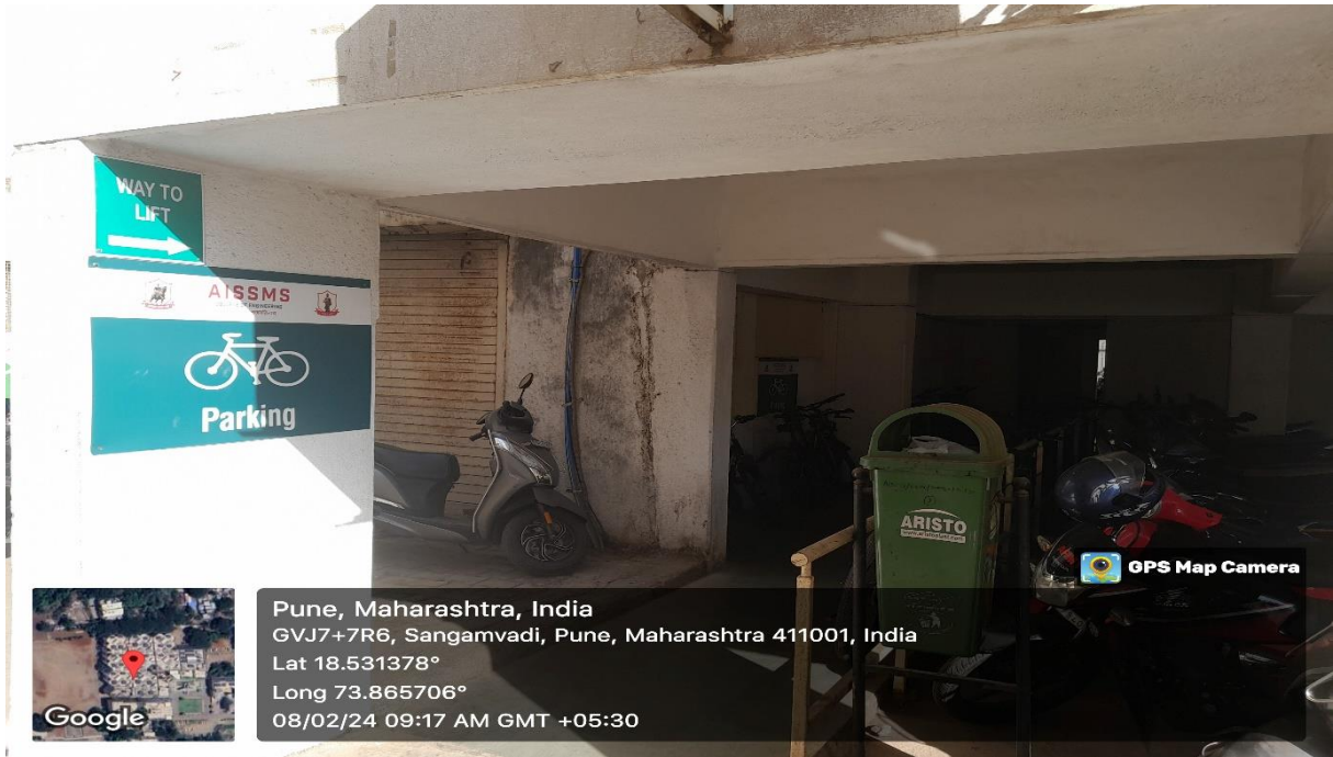
Way to lift at ground floor
