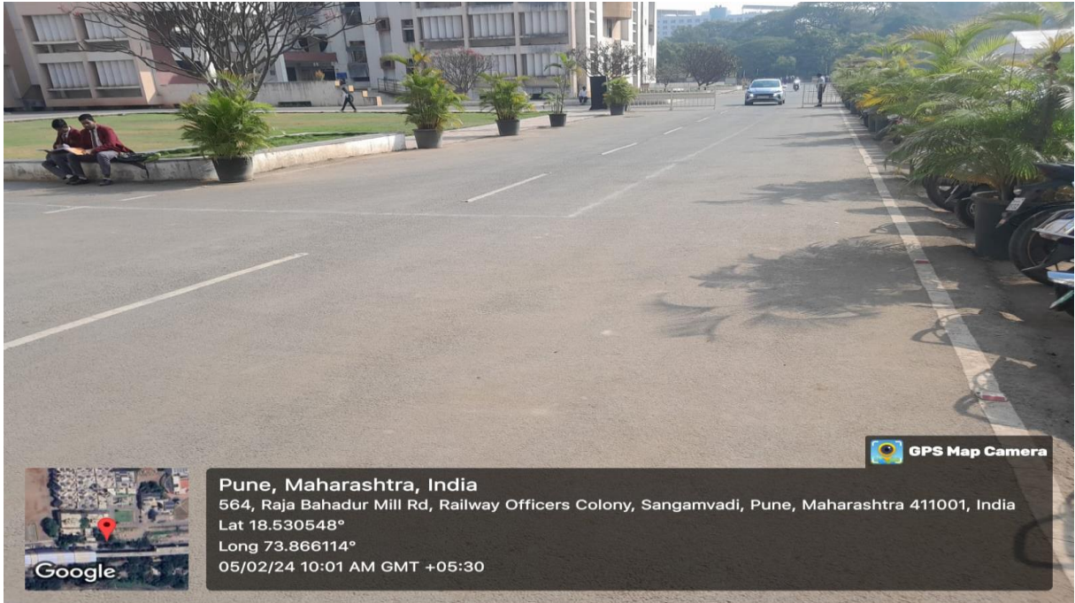
Clean and Tidy Internal Roads for Vehicle Movements
